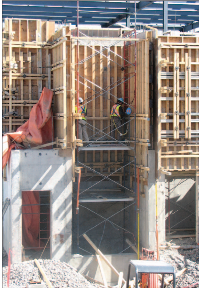
FCAS Project, shaft wall construction
