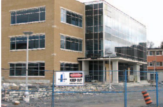
Regional Detention Centre HeadQuarters Project - Fuller Construction
