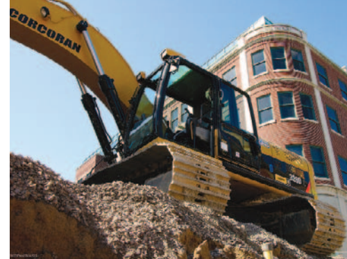
Downtown Kingston "Big-Dig" Project
