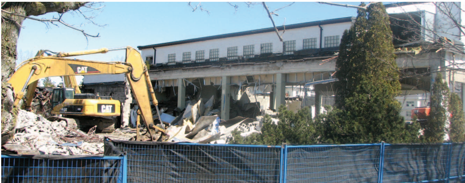
CFB Kingston demolition, Making way for new and updated facilities
